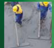
Cementing and concreting
